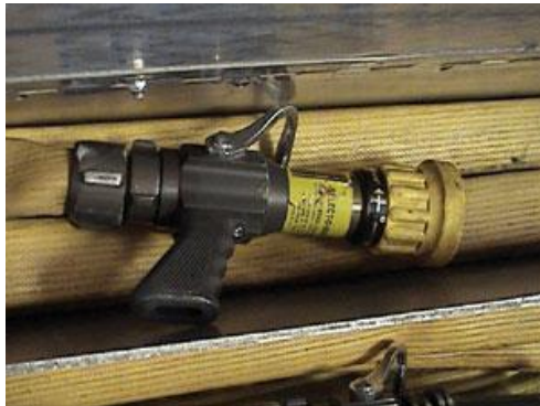
(1) The 1 \frac{3}{4} -inch automatic fog nozzle in use in Clearwater (FL) Fire and Rescue. (Photos by author.)
